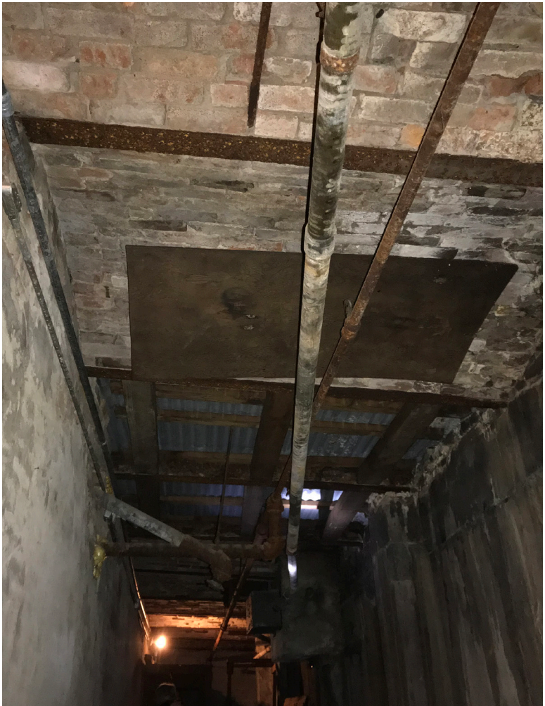
GRAND CENTRAL - AREAWAY CONDITION
